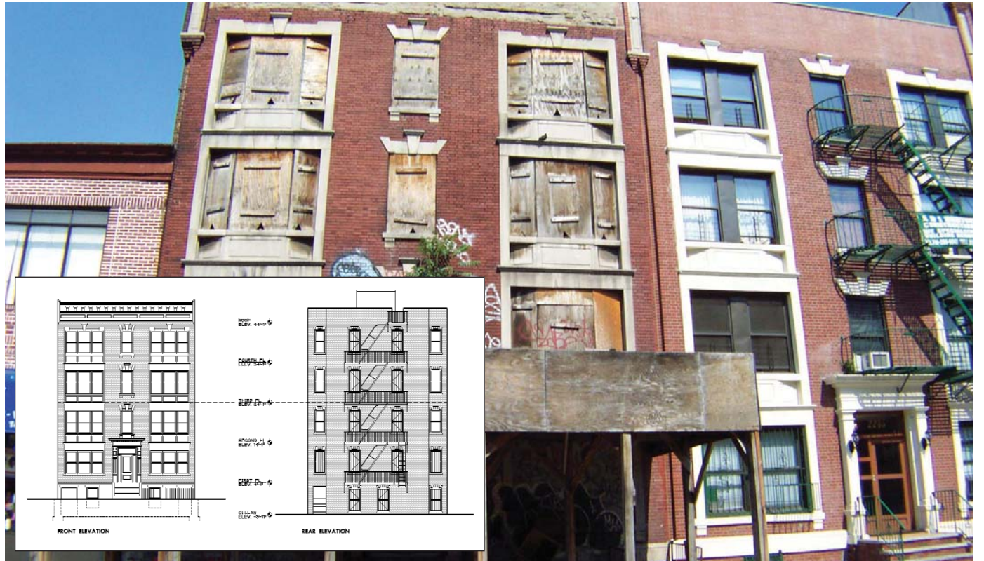
2241 Webster Avenue is a vacant nine-unit, city-owned building in the Bronx that will receive a gut rehabilitation to become eight, two-bedroom and one, one-bedroom units. Jack Coogan of Oaklander, Coogan and Vitto created the inserted elevation.
